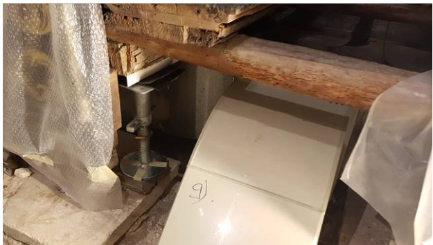
Figures 9a, 9b and 9c: Ducting very neatly accommodated beneath the choir stalls, and the custom-made ducts produced to travel beneath the Main Altar.
