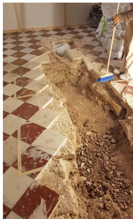
Figures 14a and 14b: Images showing the delicate removal of material to prepare the route for the required duct work. The route linked up all the four oculi.
