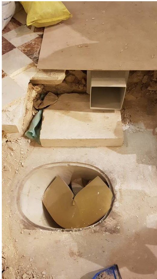
Figures 18a and 18b: The oculi exposed at Main Altar level, together with the 'original' cangatura and finished floor level. The carefully removed volume to accommodate the duct was then carefully backfilled
