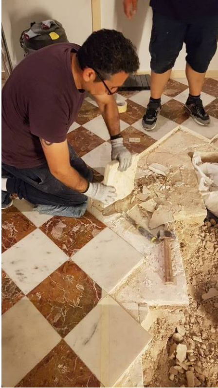
Figures 13a, 13b and 13c: Marble tiles duly marked and very carefully removed
