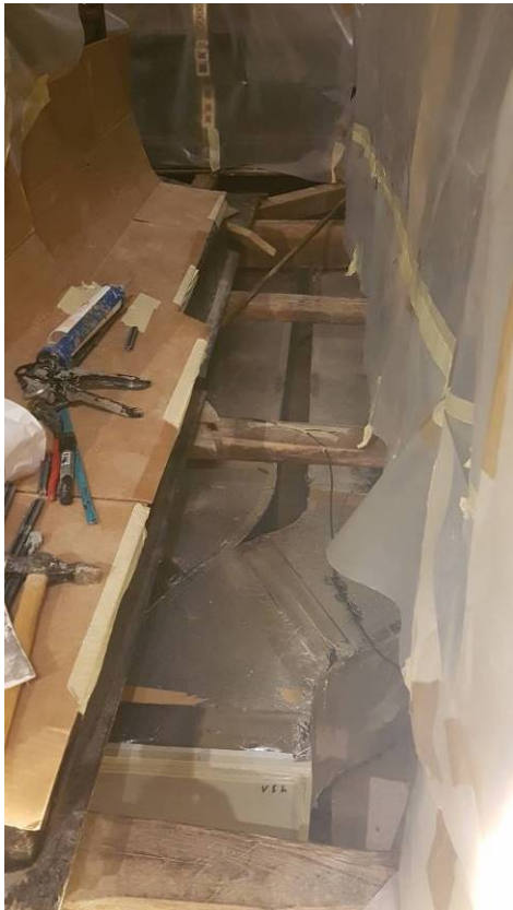
Figures 9a, 9b and 9c: Ducting very neatly accommodated beneath the choir stalls, and the custom-made ducts produced to travel beneath the Main Altar.
