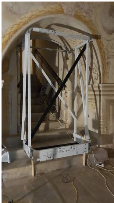
Figure 24: Image of a full scale model of the viewing gallery/platform, being fitted on site, to assess the contact points, thus ensuring that no damage is caused to the existing masonry fabric. The actual gallery/platform, which will include curved glass will be installed towards the beginning of 2019.
