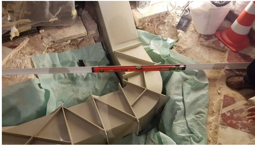
Figure 15: Detail of the custom made ducting within the routes created
