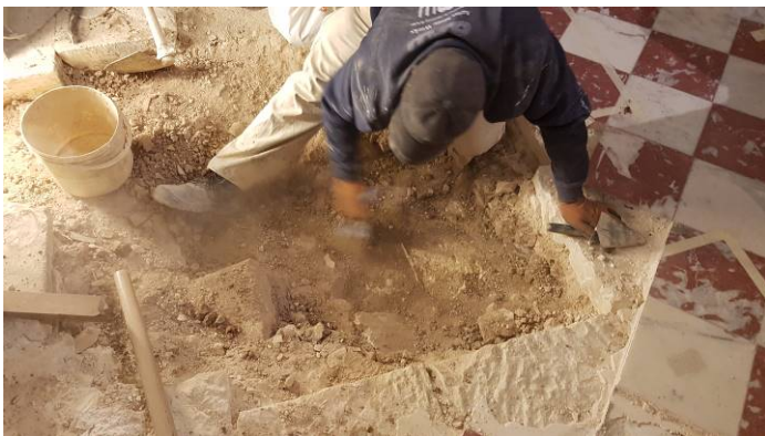
Figures 14a and 14b: Images showing the delicate removal of material to prepare the route for the required duct work. The route linked up all the four oculi.
