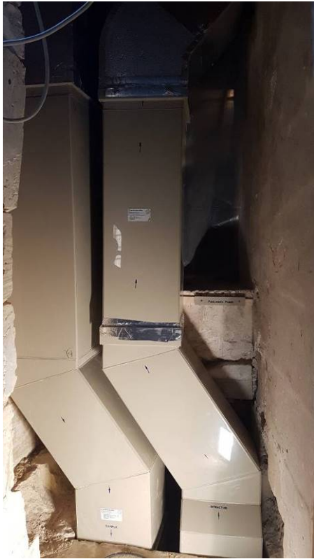
Figures 8a and 8b: Ventilation ducts tucked away neatly within the existing restricted spaces
