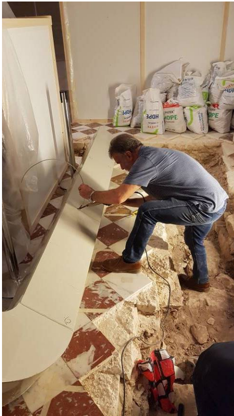
Figures 16a & 16b: Custom made ducts being manufactured on site to fit within the restricted & awkward spaces.
