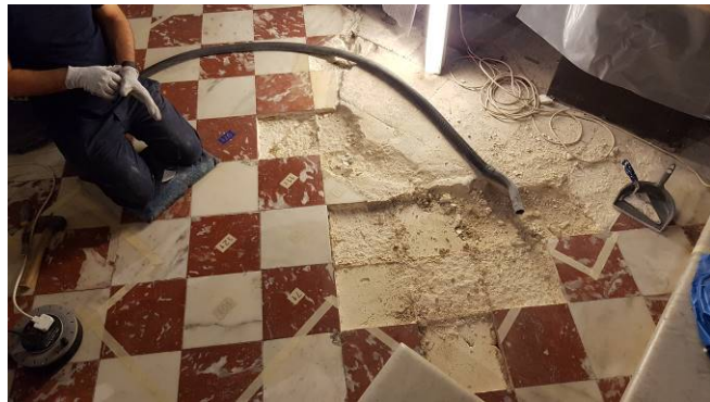
Figures 13a, 13b and 13c: Marble tiles duly marked and very carefully removed
