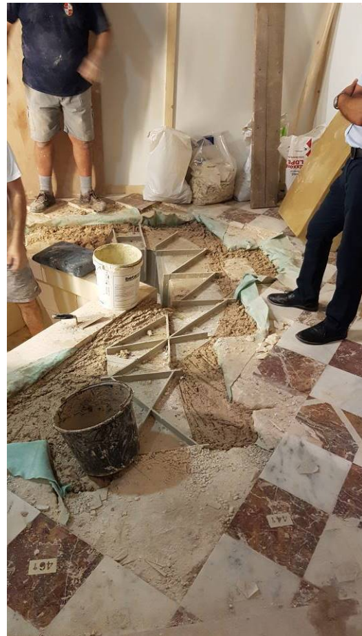
Figures 18a and 18b: The oculi exposed at Main Altar level, together with the 'original' cangatura and finished floor level. The carefully removed volume to accommodate the duct was then carefully backfilled
