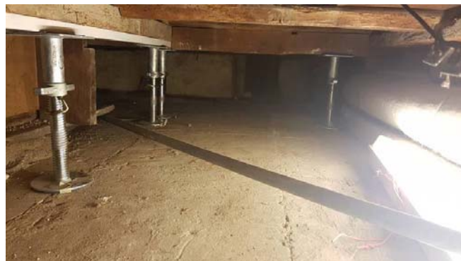
Figure 7: New structural steelwork elements beneath the choir stalls to free up the space required for the ducting
