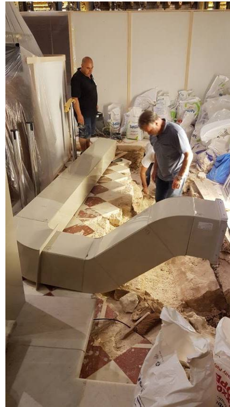
Figures 16a & 16b: Custom made ducts being manufactured on site to fit within the restricted & awkward spaces.
