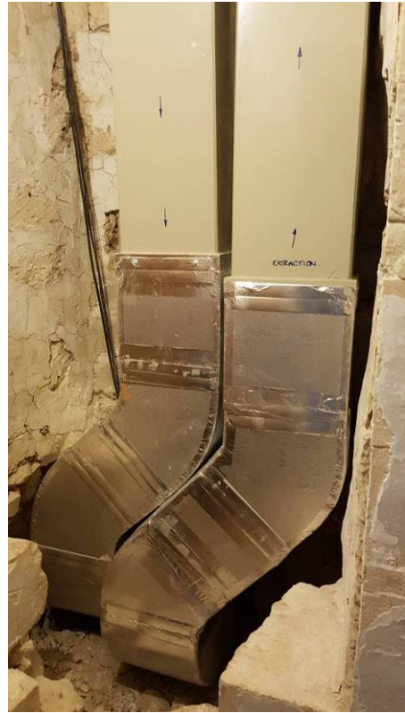
Figures 8a and 8b: Ventilation ducts tucked away neatly within the existing restricted spaces
