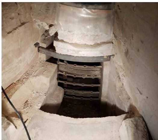
Figures 21a and 21b: Elements forming the 'original security bars, and windows jambs uncovered.
